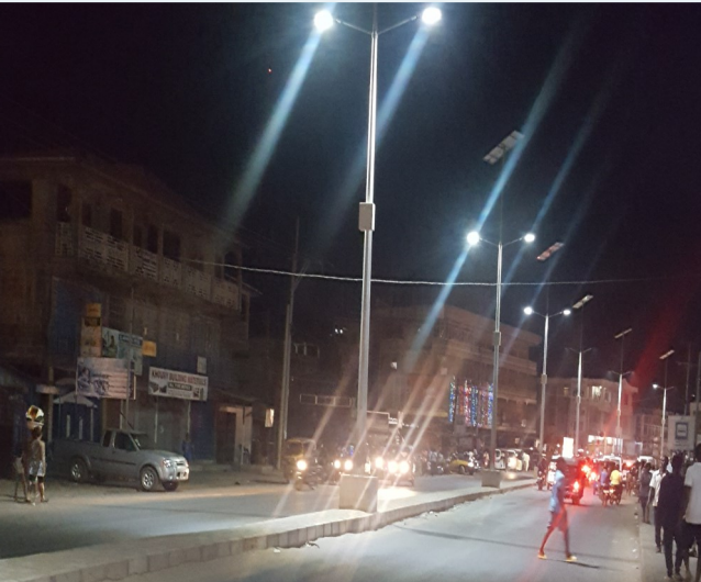
Boosting Infrastructure: NaMED together with SLRA monitored the newly constructed Imatt/ Regent road and the solar light at the Lumley main motor road for efficient result
