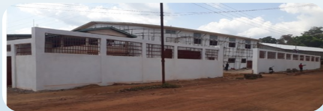
NaMED Infrastructure team together with Local Council monitored the Kenema City Hall for rapid completion of quality result
